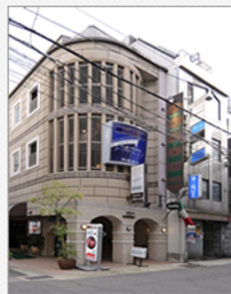
Nuova Spirito Bldg 3rd Floor
